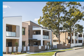
An example of the new social housing built in Lugarno
